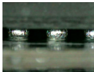
Cracks Wide View
